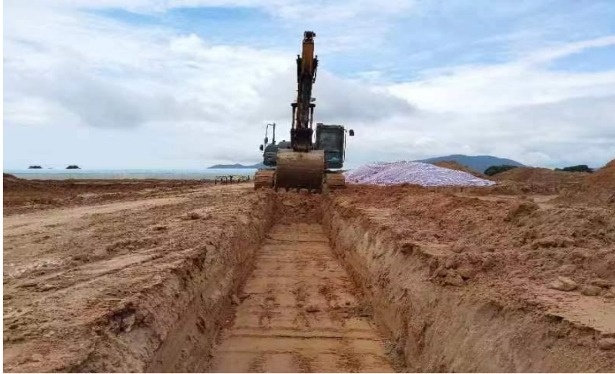
斗沟沟槽开挖
