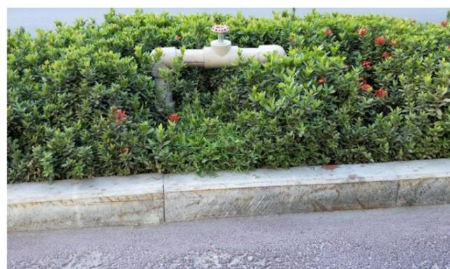
隔离带路缘石，石面破损，石面有槟榔渍
